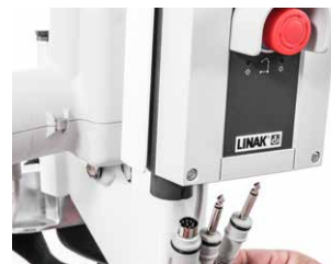
Checking wires connection
