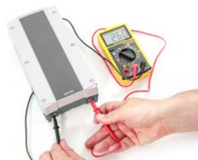
Checking voltage on battery
