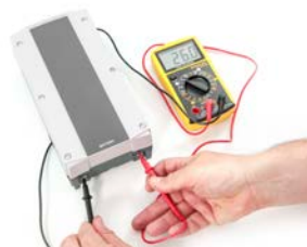
Checking voltage on battery
