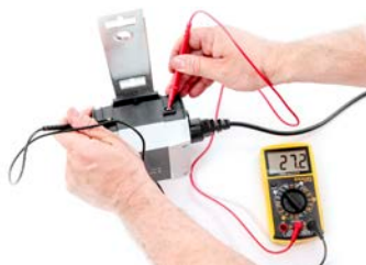
Checking voltage on charger
