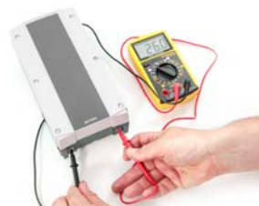
Checking voltage on battery
