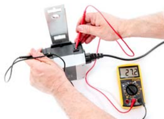
Checking voltage on charger
